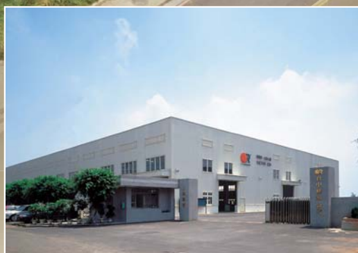
Industrial park factory : 21110 m 2 (PIM machinery)
